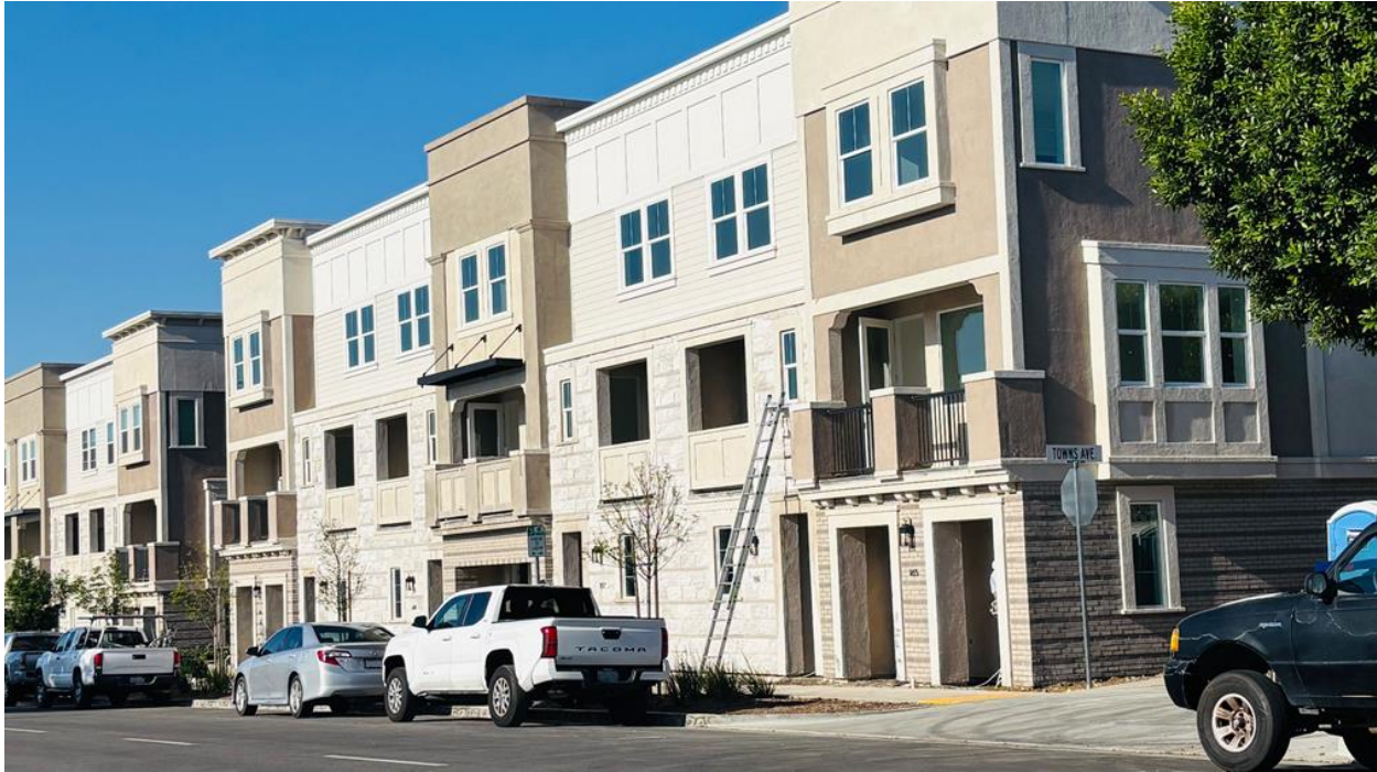
Towns on First - Building 4 - First Avenue/A Street (Under Construction) - May 2026
